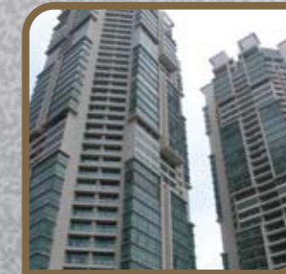
Marc Service Residence
